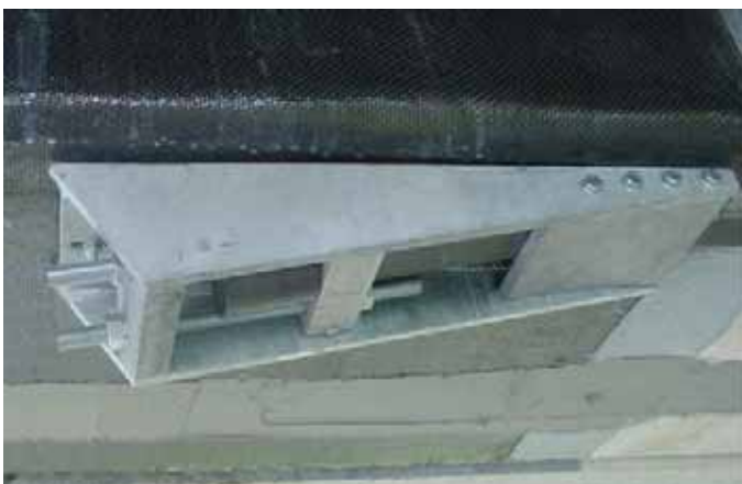
ill. 8: ancrage mobile type III
