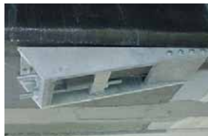
III. 2: ancrage mobile type III
