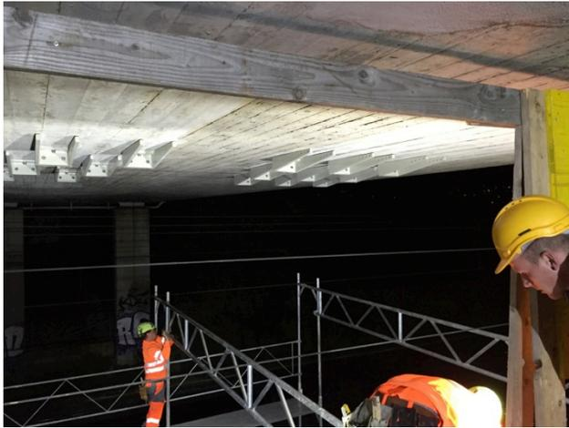
Figure 01: Mobile scaffolding structure
